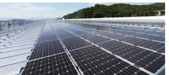
generator reading of photovoltaic system can be checked on a monitor in the entrance hall. All generated energy is sold and it contributes to power supply of local area. Installing solar panels mitigates the rise in temperature inside of the plant, so that it could also reduce energy cost of air-conditioning in summer.
